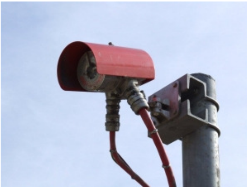
Sample Image of Flame Detector installed on a parking lot pole 5
