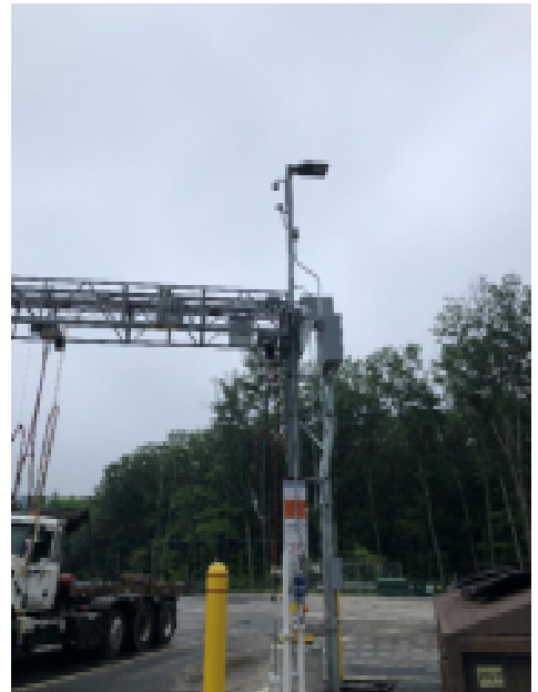
Sample Image of Flame Detector installed on a parking lot pole 5
