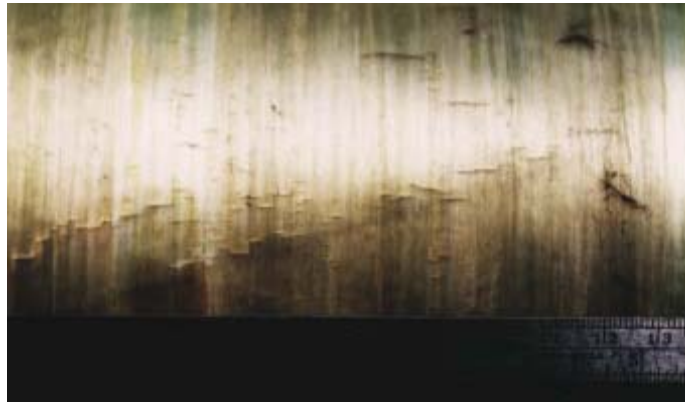
Figure 5.2 Stress Corrosion Cracking (SCC)
